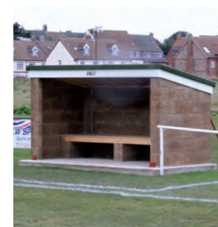
The new team shelters at Wells Town FC
